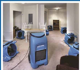
Structural Drying
